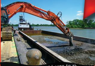
2) Transported barge to the mixing/unloading site and solidified the material by adding blown lime.
